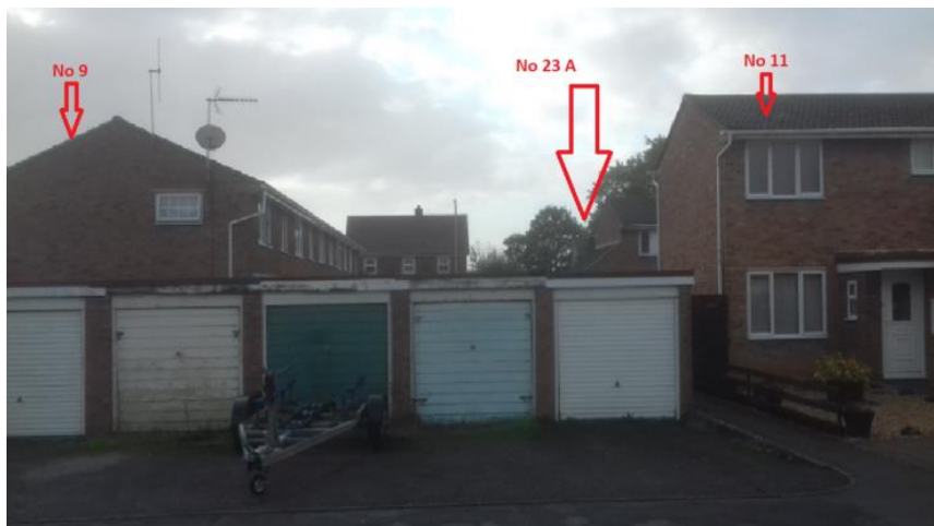
View of No 9 and No 11 Baydon Close with No 23a in the background
